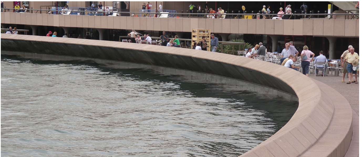
Galvanized Reinforced Sea-wall – Sydney Harbour
