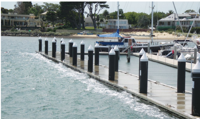
Galvanized Reinforced Wave-wall – Port Phillip Bay
