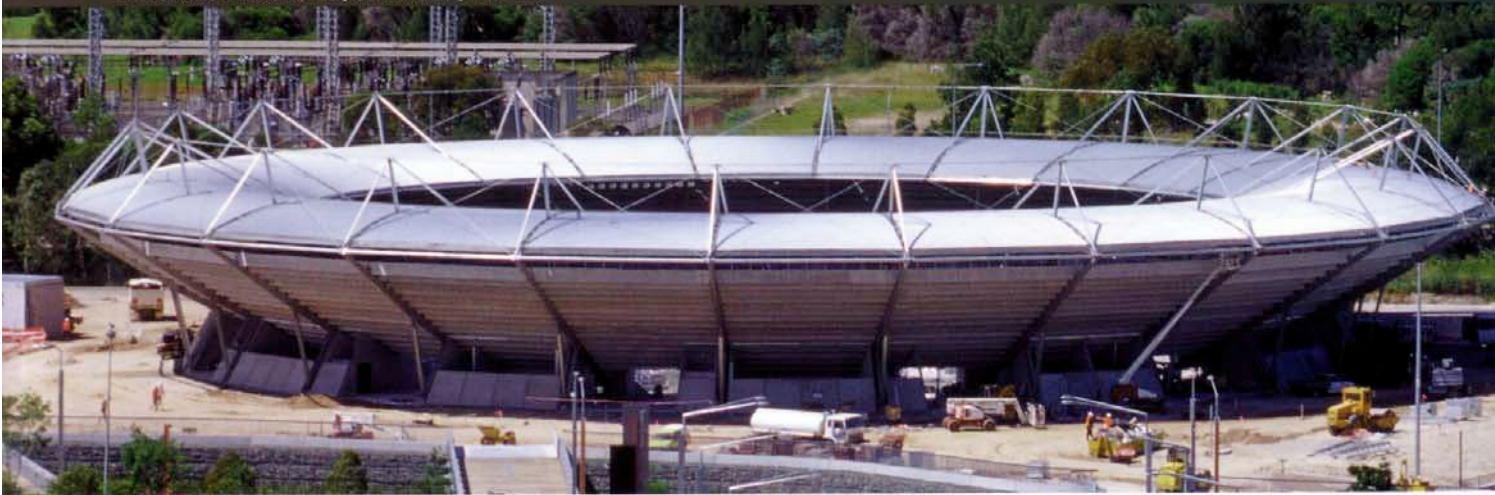
NSW Tennis Centre, Homebush Bay (Photographs courtesy of Bligh Valler Nield)
