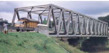
Standard Truss Bridging
