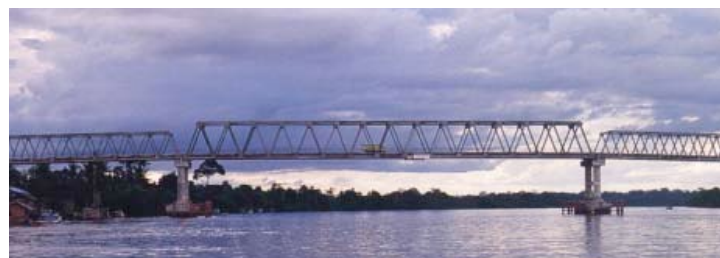
Long Span Truss Bridging
