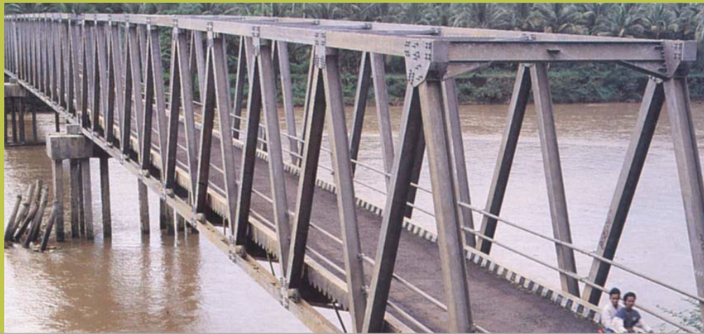
Single-Lane Permanent Span C-Class Truss, multi-span
