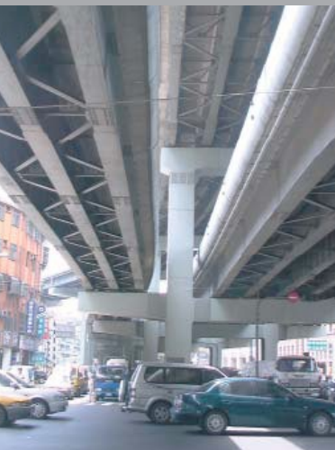
Chung Cheng Overpass, Taiwan
