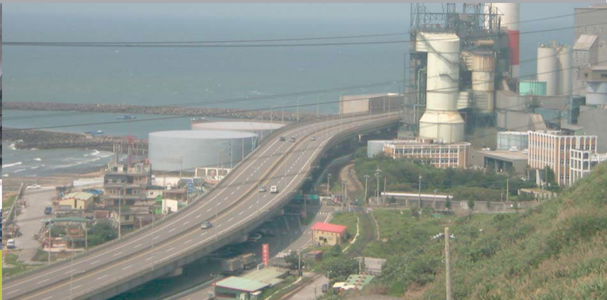
Chung Cheng Overpass
