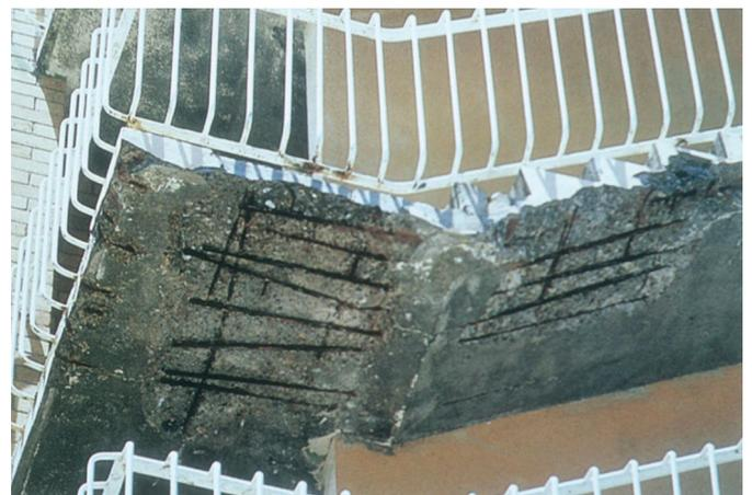
Deterioration of the bare steel reinforcement in a coastal balcony
